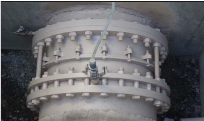
Fig. 5 - 30" wafer mixer installed between flanges
